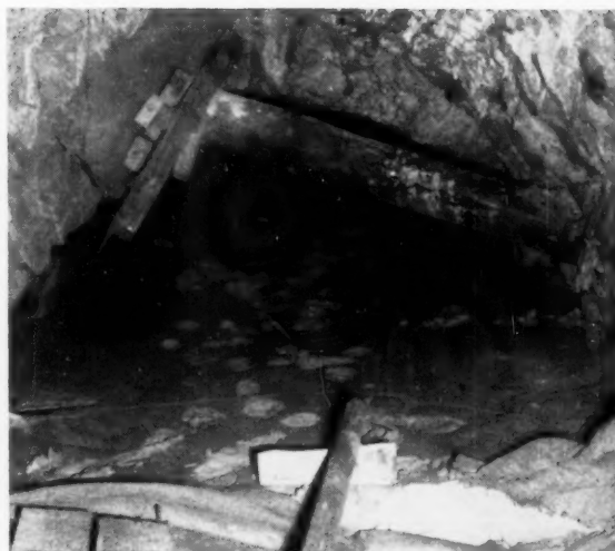
AFTER FILLING stope with sand through pipe at bottom, four to six hours are needed before it solidifies. About 5,000 tons of sand fill are placed monthly in the mine.
